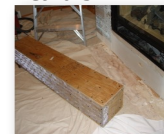
Wire Mesh applied over drywall.
