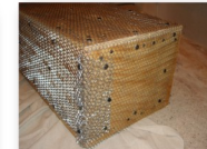
Scratch-coat of mortar applied.
